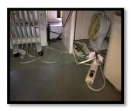
Here again, most model codes and manufacturers have very specific requirements: electric heating appliances must be plugged directly into a permanently installed wall receptacle—not into an extension cord and not into a reloacatable power tap. Under optimal
