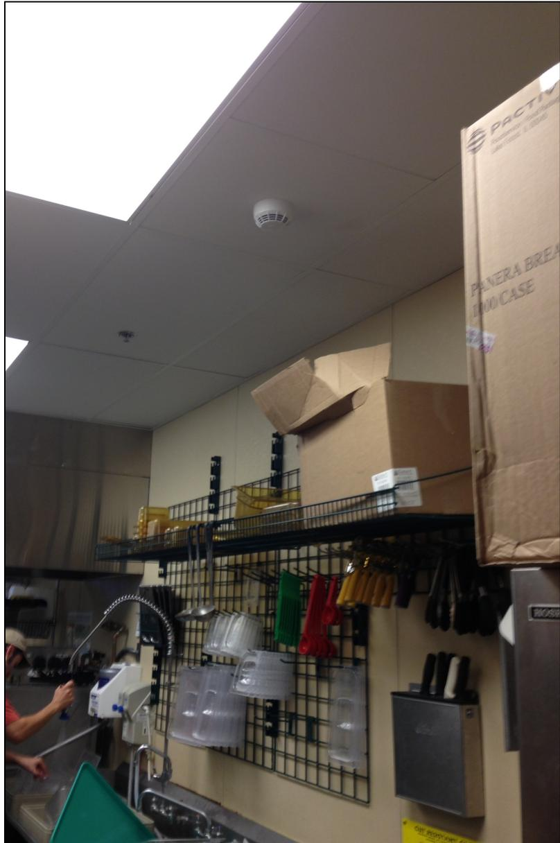
*The smoke detector installed in the restaurant dish room that generated numerous unwanted alarms.*
