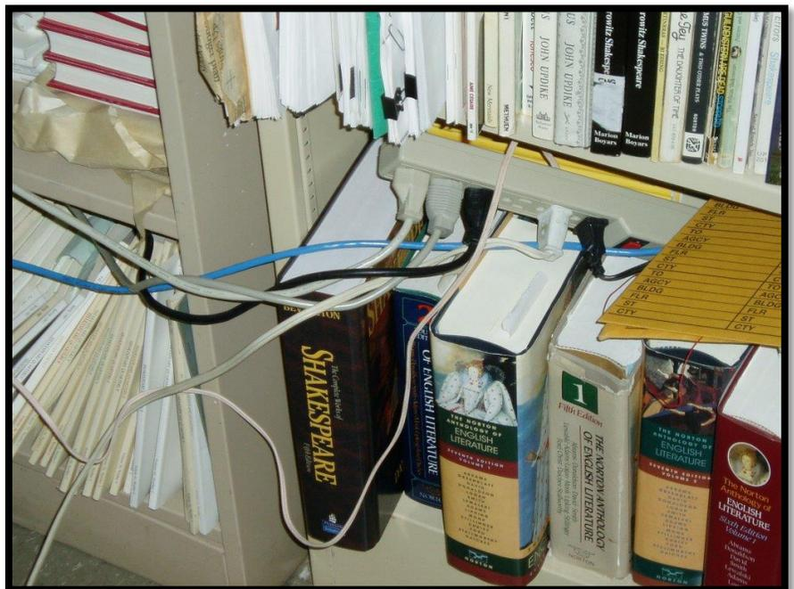
conductors and replace it with a \$5.00 dollar plastic device of questionable provenance. It may possibly be a legitimately listed device, although counterfeits are common, but more than likely it is not protected against
